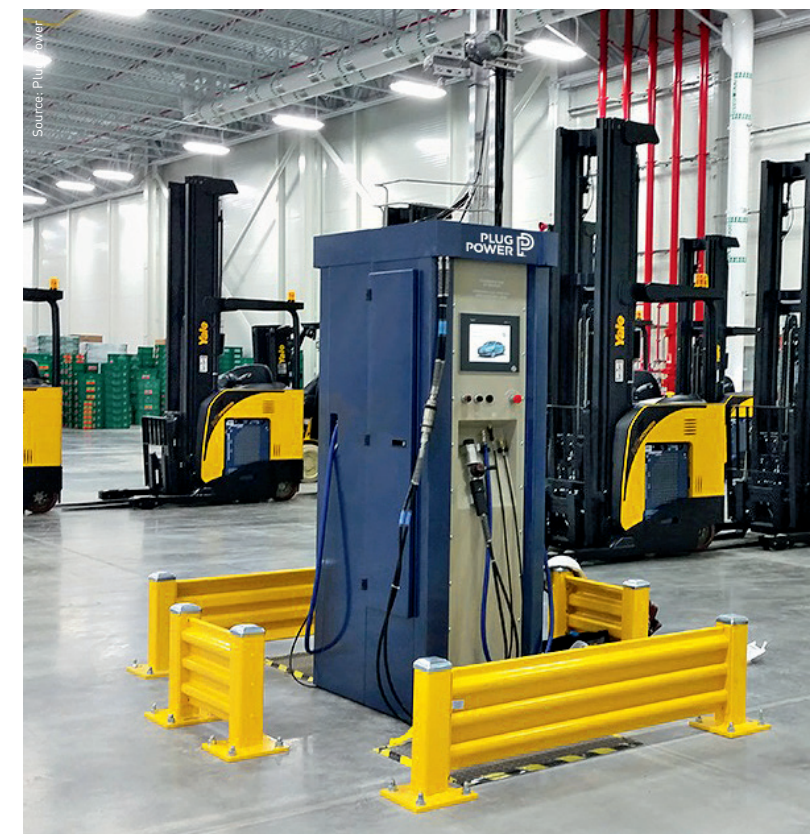
Fig. 3: H 2 refueling station in warehouse
