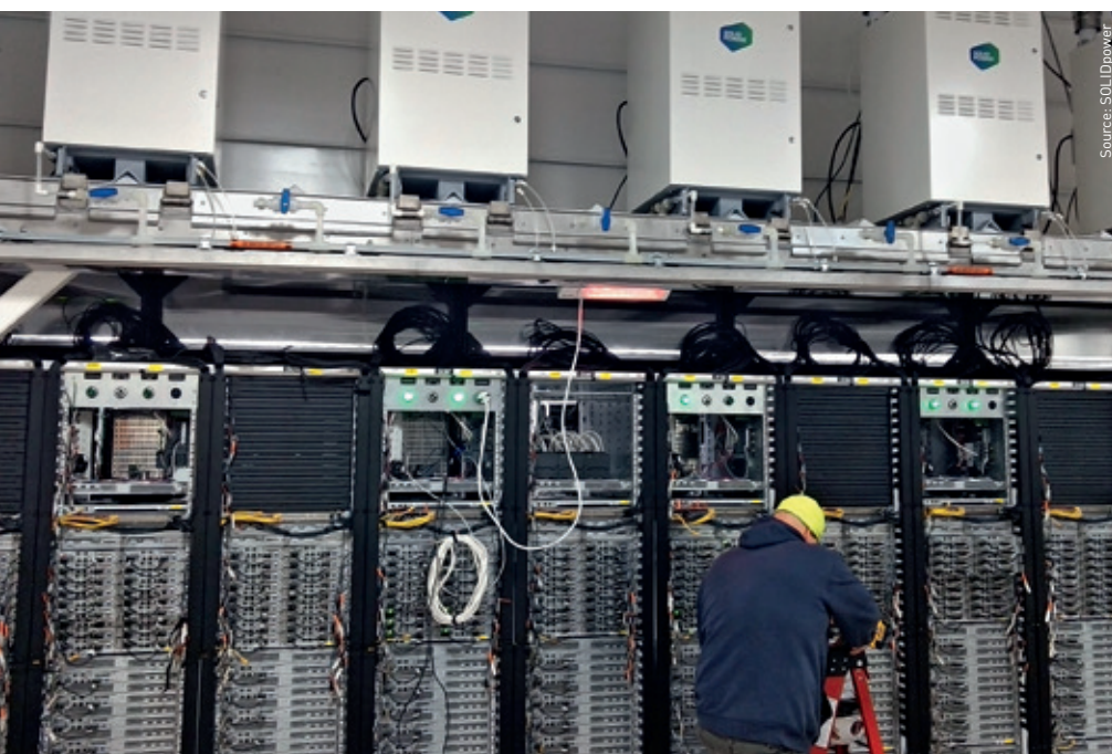
Fig. 2: Fuel cell units on top, servers directly below
