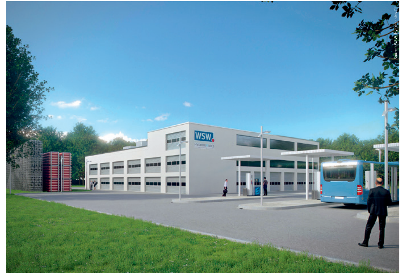
Fig. 1: Hydrogen refueling station with on-site electrolyzer; maximum production rate: 6 tons / day
