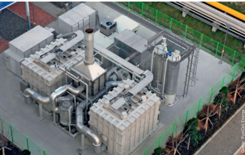
Fig. 3: SureSource 3000, consisting of two 1.4-megawatt units
