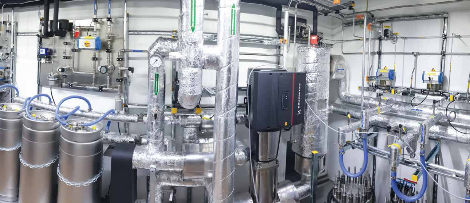
Fig. 6: View inside the 500-kilowatt Green Electrolyzer [Source: iGas]
