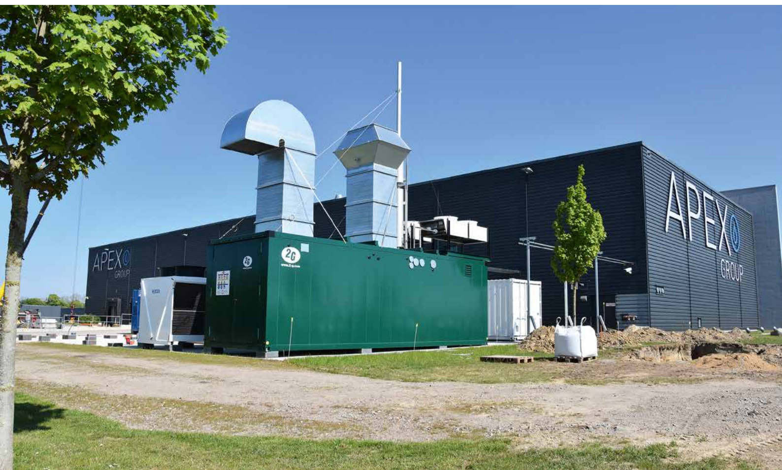
Fig. 3: Structure of hydrogen power plant with an H 2 -CHP unit from 2G at Apex
