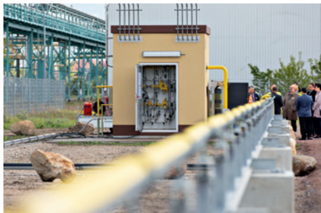
Fig. 1: System components of the H_2 infrastructure: above-ground pipe bridge and gas pressure regulator station [Source: Michael Setzpfandt]
