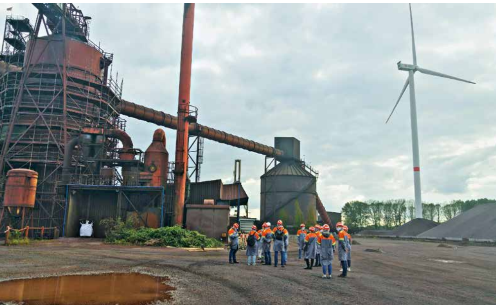
Fig.: In the Midrex plant (left), ArcelorMittal obtains iron through direct reduction. Its successor is expected to one day use hydrogen instead of natural gas. [Image: Eva Augsten]
