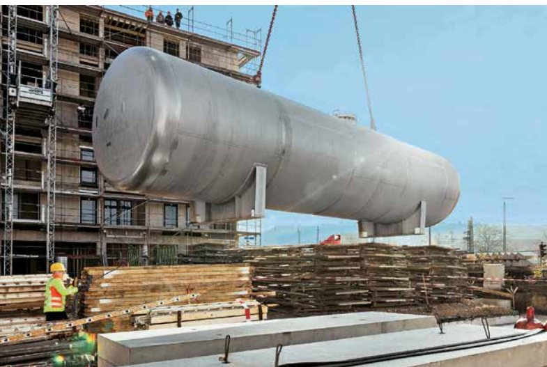
Fig. 2: Installation of the 32-foot-long [10-meter] hydrogen tank in Esslingen [Source: Neue Weststadt]
