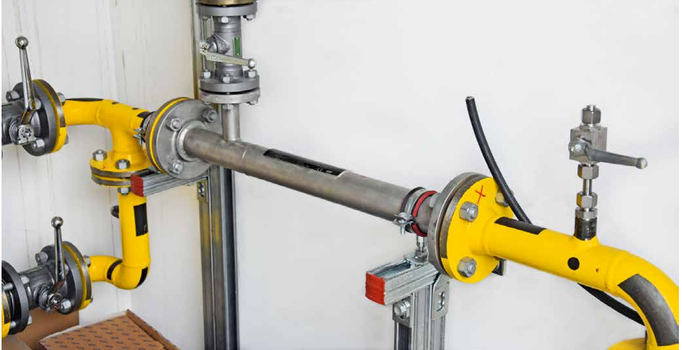
Fig. 4: The gas mixer is a rather inconspicuous piece of pipework
