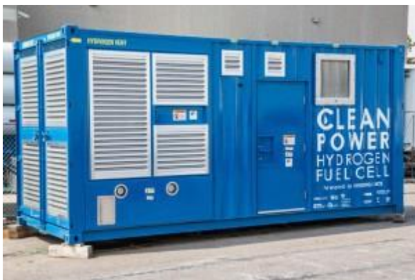
PEM-electrolyzer in a container (Source: Hydrogenics)
