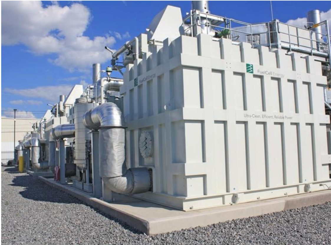
Fuel cell power plant, © FuelCell Energy
